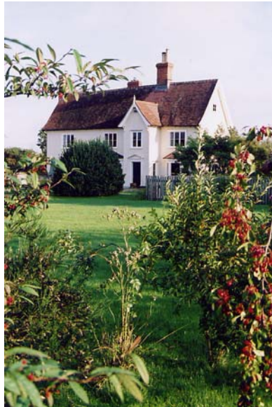
Church Farm, Gosbeck - After timber frame repairs, remodelling and refurbishment
