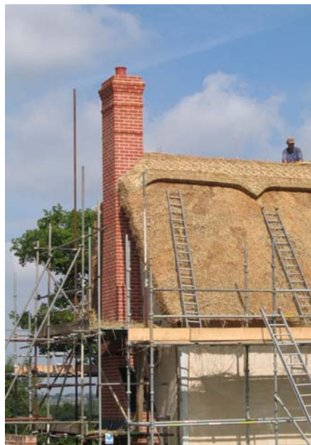
Grove Farm, Brandeston - extension and restoration
