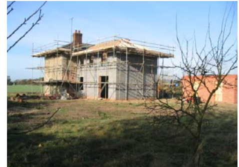
Peyton Hall, Ramsholt - extension under construction
