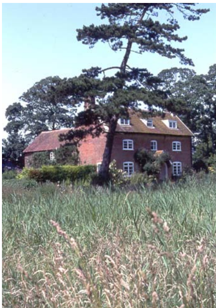
Poplar Farm, Ramsholt - restoration and refurbishment
