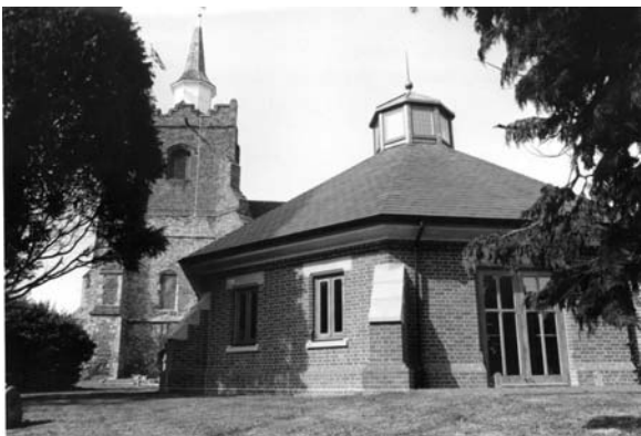
St. Mary's Church Hall, Maldon. The new hall overlooks the Blackwater Estuary. The octagonal pavilion was designed to provide a meeting hall, with ancillary facilities including kitchen, choir vestry and parish office. The octagonal form with its bold buttresses takes the character of a traditional Chapter House, and the stone dressing of the offsets, and projecting eaves appropriately suggest Gothic forms.
