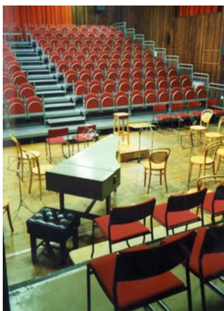
The Jubilee Hall, Aldeburgh. Various repair and improvement projects, including retractable seating, new entrance, facilities for the disabled and fire precautions work.
