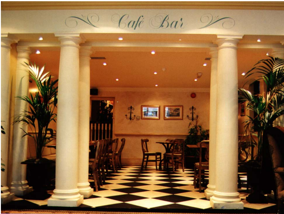
Interior view of entrance into Café Bar. New Columns are purpose designed and formed in fibrous plaster.
