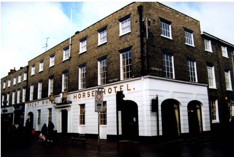
New front elevation showing remodelling of ground floor façade, reinstating the sash windows and providing new entrances to the bar area's.
