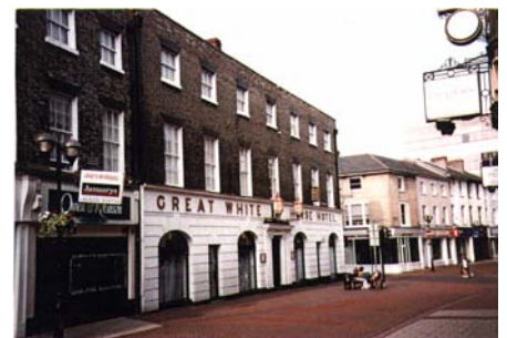
Tavern street frontage before alterations.
